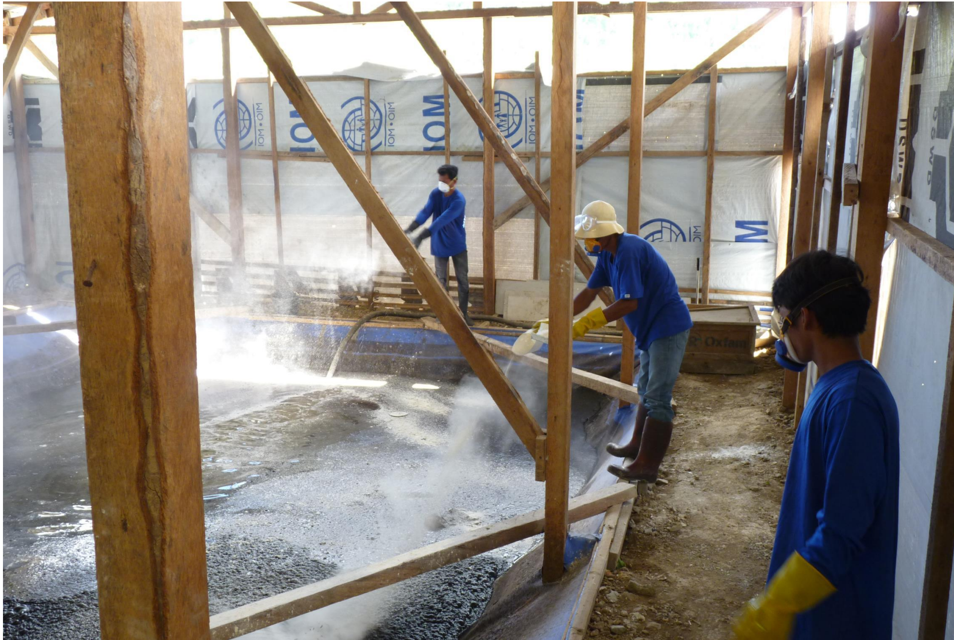
Lime application on a faecal sludge storage pond
