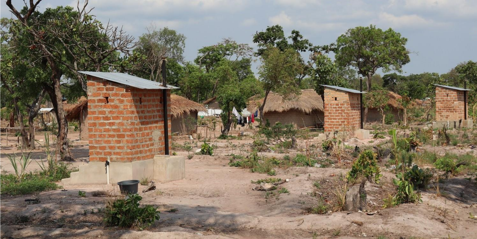
Raised latrines in Mantapala, Zambia (Ph. Reymond, UNHCR)
